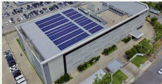
Solar panels were installed on the roof of our R&D Center in Thailand
