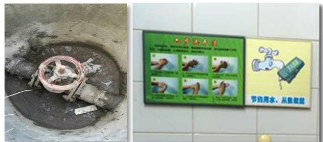
Valve mounted on branch water pipe in Fujitsu General Central Air-Conditioner (Wuxi)
