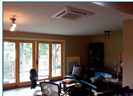
A compact cassette was installed in the upstairs living room while wall mounts were installed in the newly created bedrooms on the lower level.
