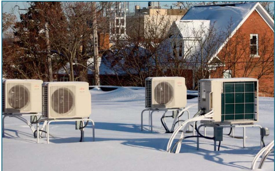
*The historical look of the building and isolation of equipment was achieved by installing the majority of outdoor units either on the roof or indoors, in 3 separate mechanical rooms in the basement. This also kept the units isolated to prevent theft.*
