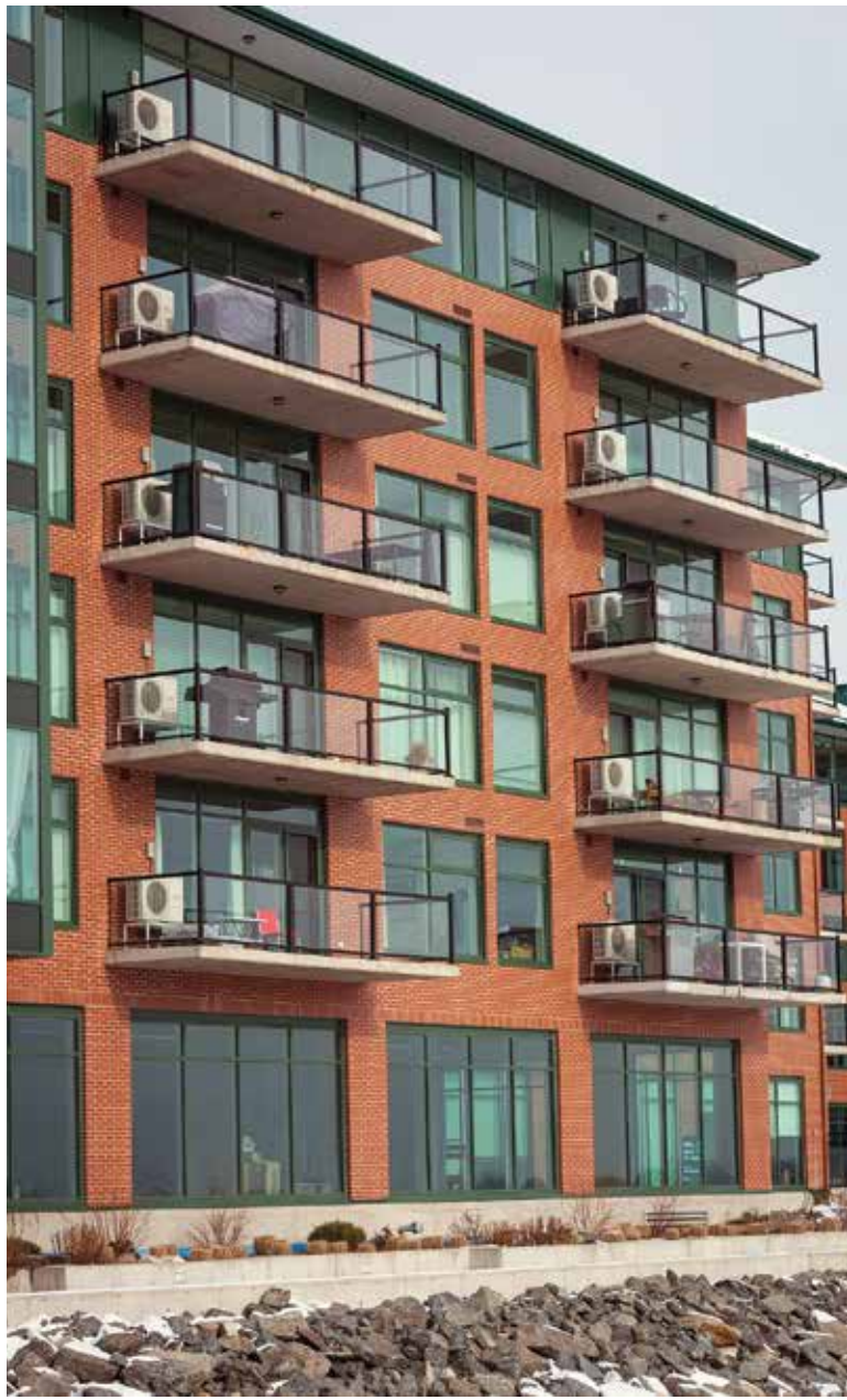
The project includes a total of 79 Fujitsu RLXFZ units for the condo units and one common area.
