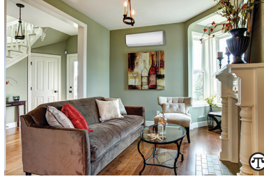
Many homeowners give a warm welcome to innovative energy- and cost-efficient HVAC systems.
