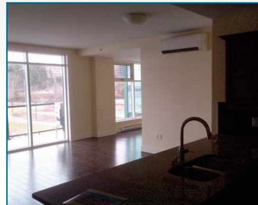
A combination of wall mounts and concealed slim ducts units were used inside the condo complex.
