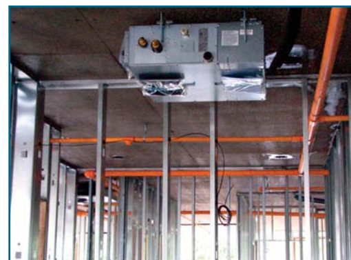
A combination of wall mounts and concealed slim ducts units were used inside the condo complex.
