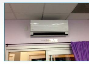
25 Wall mount systems and 2 multi-zone systems connected to 6 compact cassettes provide heating and cooling to 24 individual suites.
