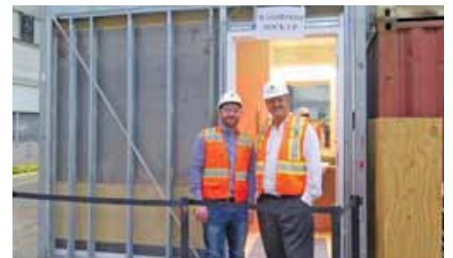
Factory-built buildings 12 Increased pre-fab drives different mechanical approach
