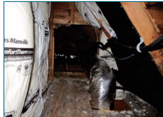
Registers from a Slim Duct unit are shown above, installed in one of the bedrooms. Below, just a minimal amount of flexible duct, the line set and electrical line run through the attic space.
