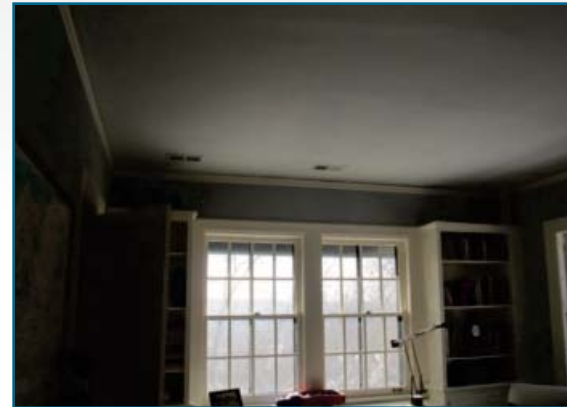
Registers from a Slim Duct unit are shown above, installed in one of the bedrooms. Below, just a minimal amount of flexible duct, the line set and electrical line run through the attic space.
