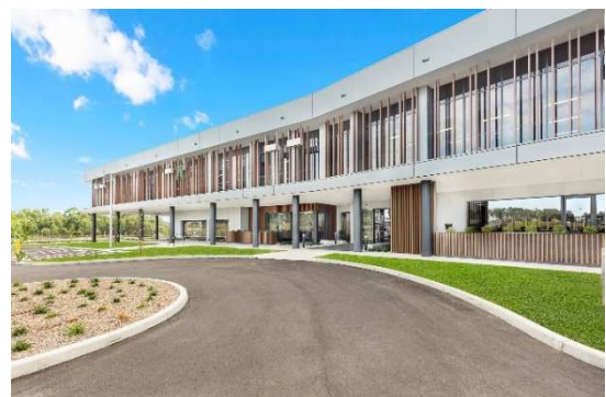
The new head office of Fujitsu General Australia in Sydney, which became operational in May 2019
