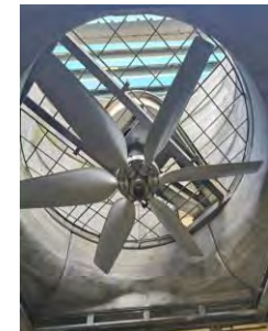
Lightweight plastic fans in cooling tower
