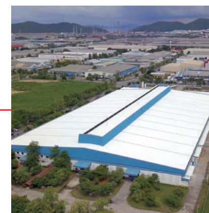
Fujitsu General (Thailand) Co., Ltd. (Thailand) Factory-2
