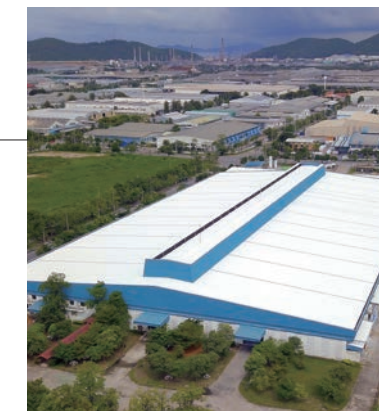
Fujitsu General (Thailand) Co., Ltd. (Thailand) Factory-2
